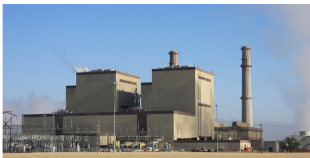
Tolk Generating Station | Xcel Energy
