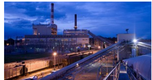
Yorktown plant | Dominion
